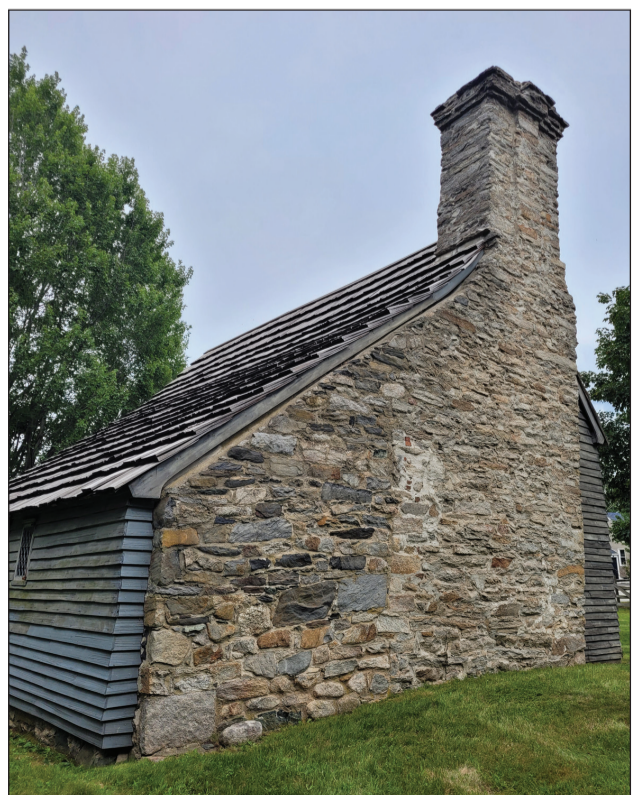
STONE-ENDER: The Clemence-Irons House is a rare surviving 'stone-ender,' a type of architecture used by New England's earliest European settlers. Most houses of this type burned during King Phillip's War.
